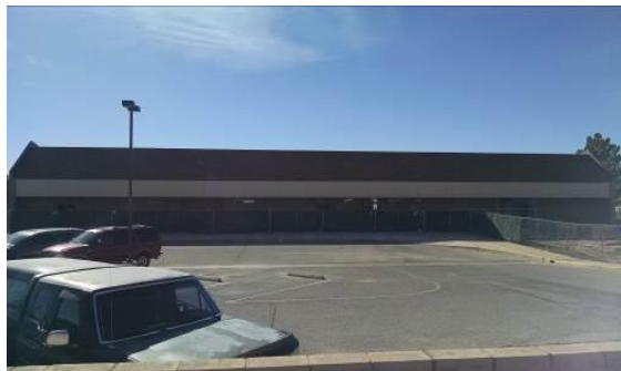
North Face of New Building
