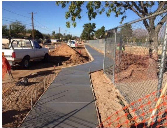
Curbing and sidewalk
